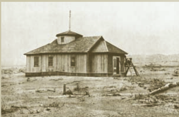
▲ “Orthodox Chapel at Katmai, 1915, showing effects of flood” Photo courtesy of National Geographic Society.
